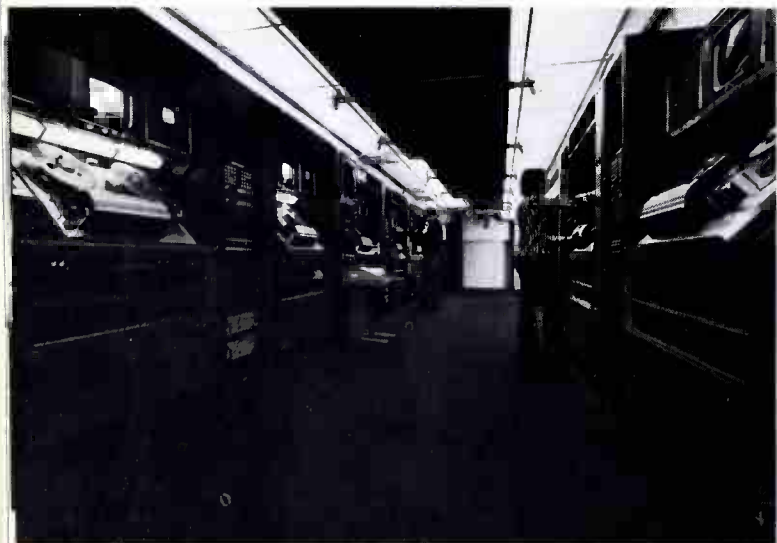
Teletronics has separated VTR equipment from the editing rooms so that the latter are quiet and distraction free.
